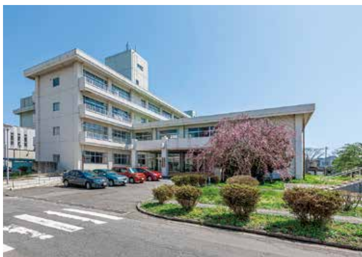
保健学科棟 Building for Health Science
