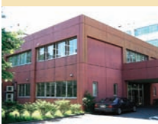
管理棟 Administration Building
